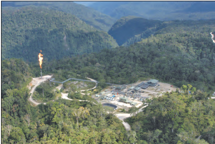
Plate 2.4 Agogo Production Facility
