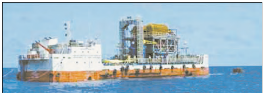
Plate 4.6 Barge-mounted desalination plant
