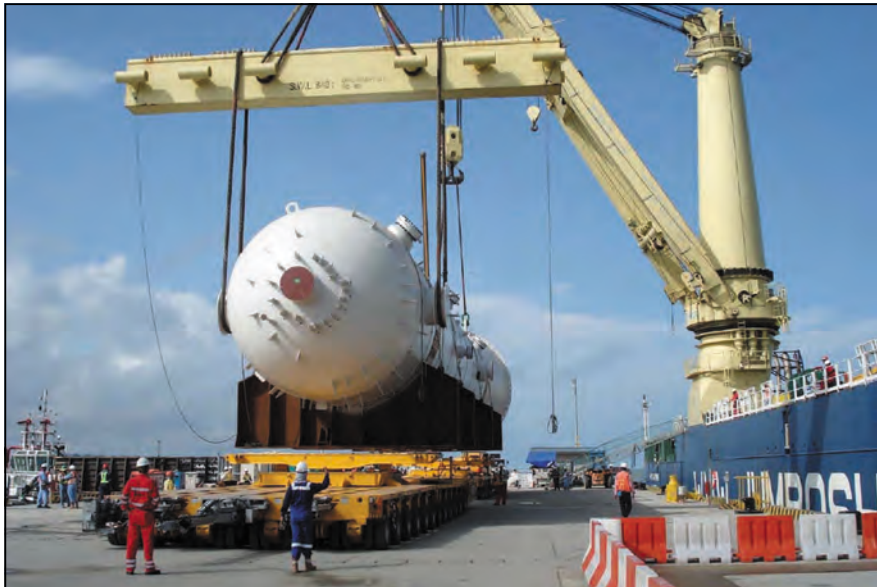
Plate 4.7 Amine absorber being unloaded
