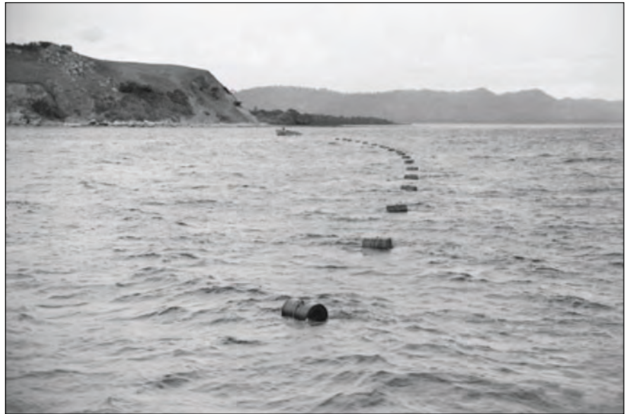
Plate 16.16 October 1943 Boera Point, New Guinea: drums with the marine telegraph cable attached being towed to shore
