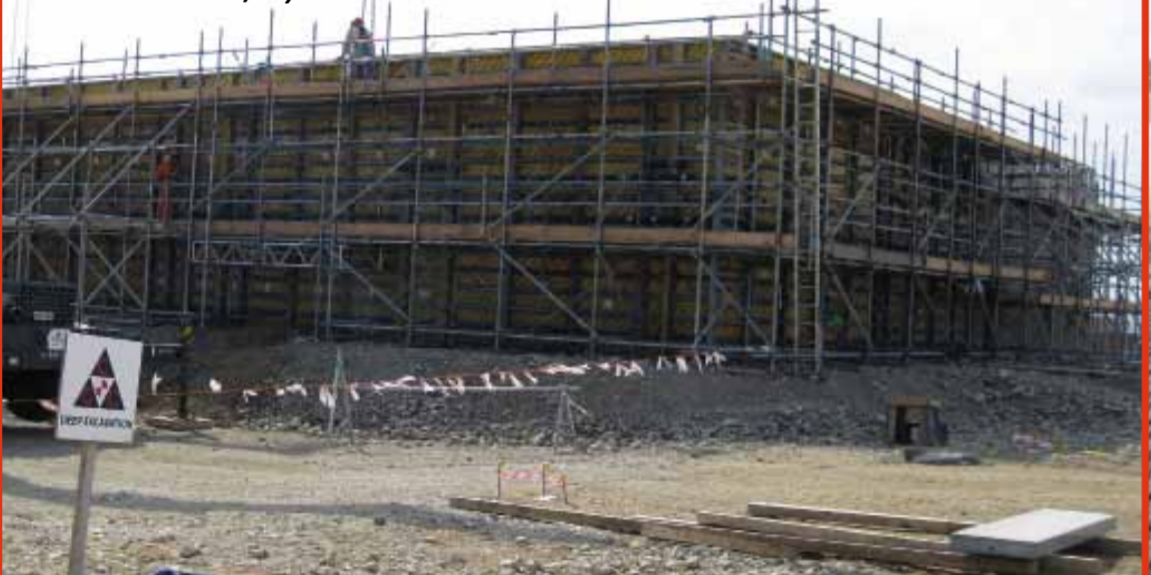
The pipe racks for the Process Trains are being built by Daewoo. These tall steel structures will carry approximately 65 kilometres of pipes and most of the systems needed to clean and cool the gas.
