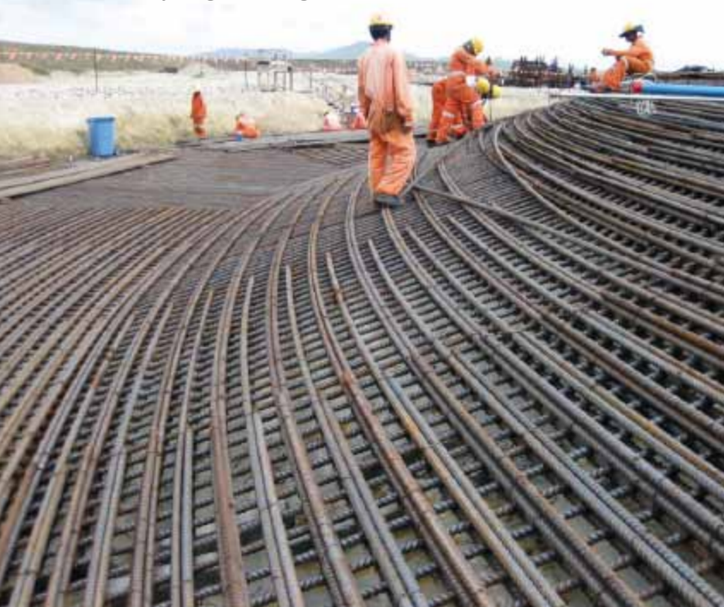
CBI workers have been welding the 1,128 tonnes of reinforcing steel for the LNG tank foundations. With 5,970 cubic metres of concrete per tank foundation, the tanks are slowly rising above the ground.
