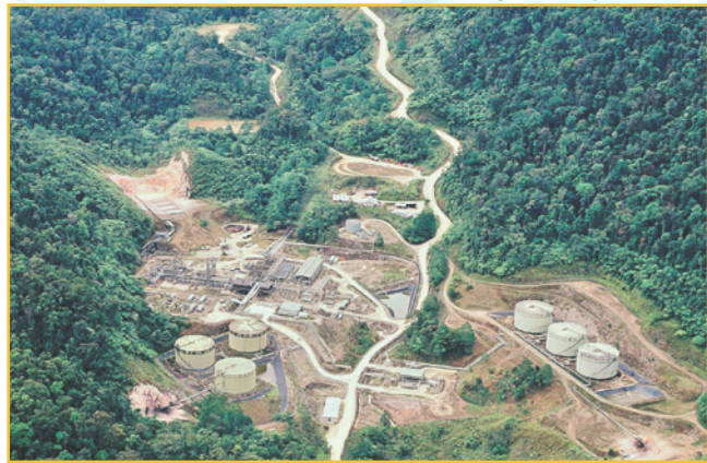
Plate A1.1: Kutubu Central Processing Facility
