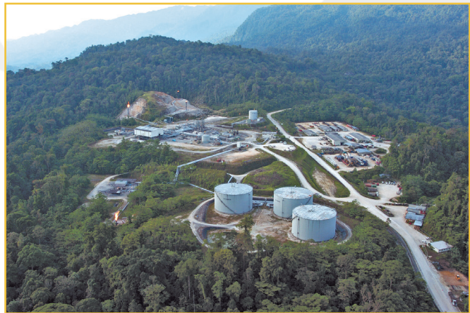
Plate 2.1: Gobe Production Facility
