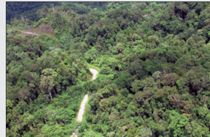
Existing controlled-access petroleum road near the Kutubu Central Production Facility
