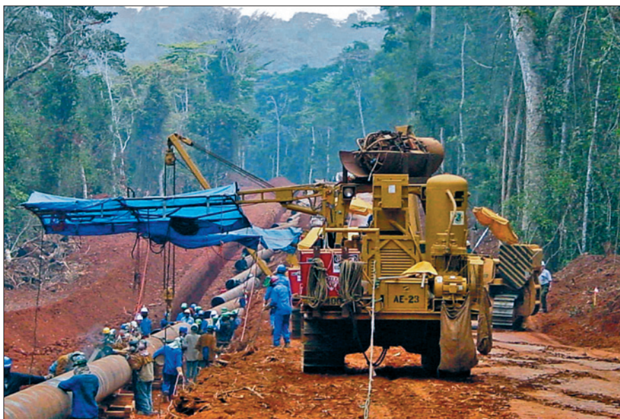
Plate 3.18 Example of pipespread stringing and welding pipe
