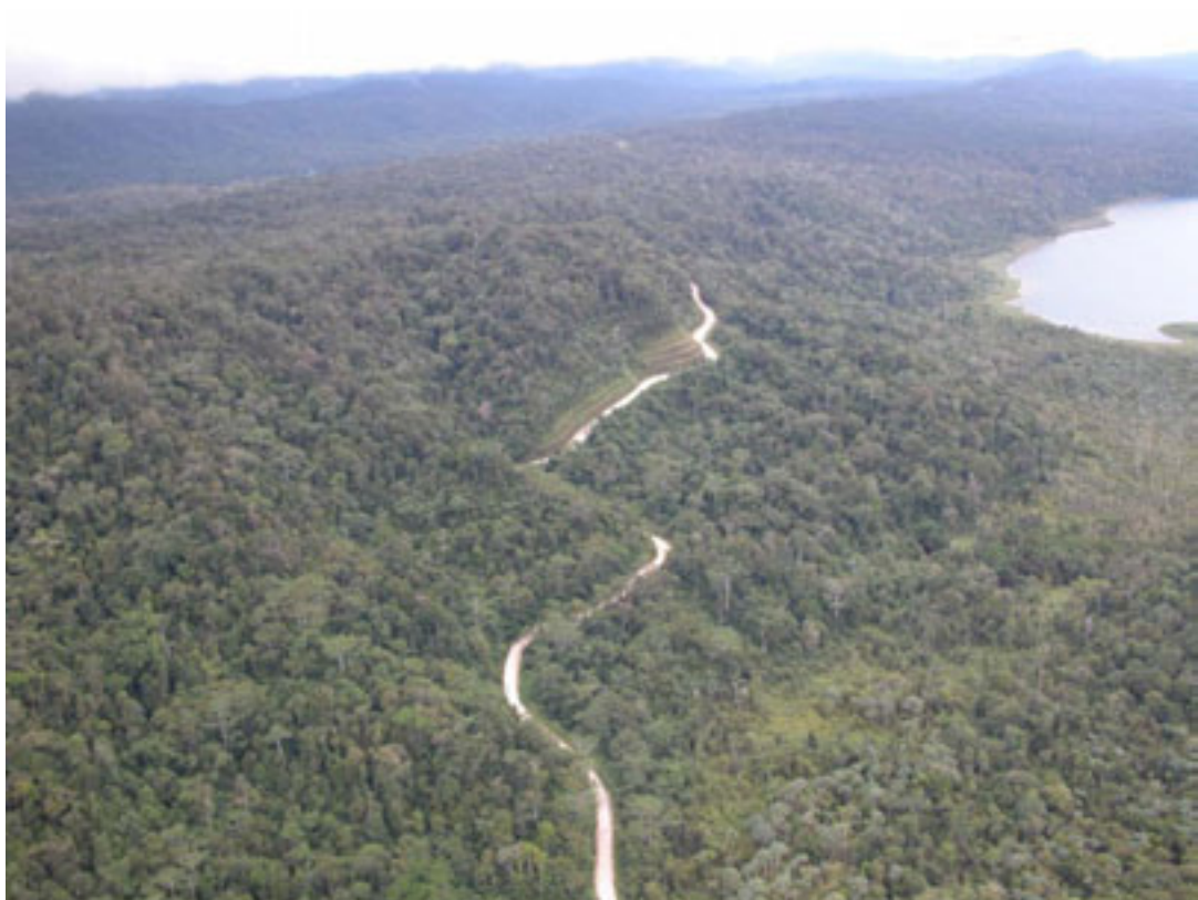
Plate 105 Cutting on road at northern end of Lake Kutubu.
