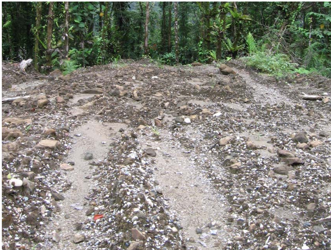
Plate 5 Example of topsoil erosion where vegetation has been cleared
