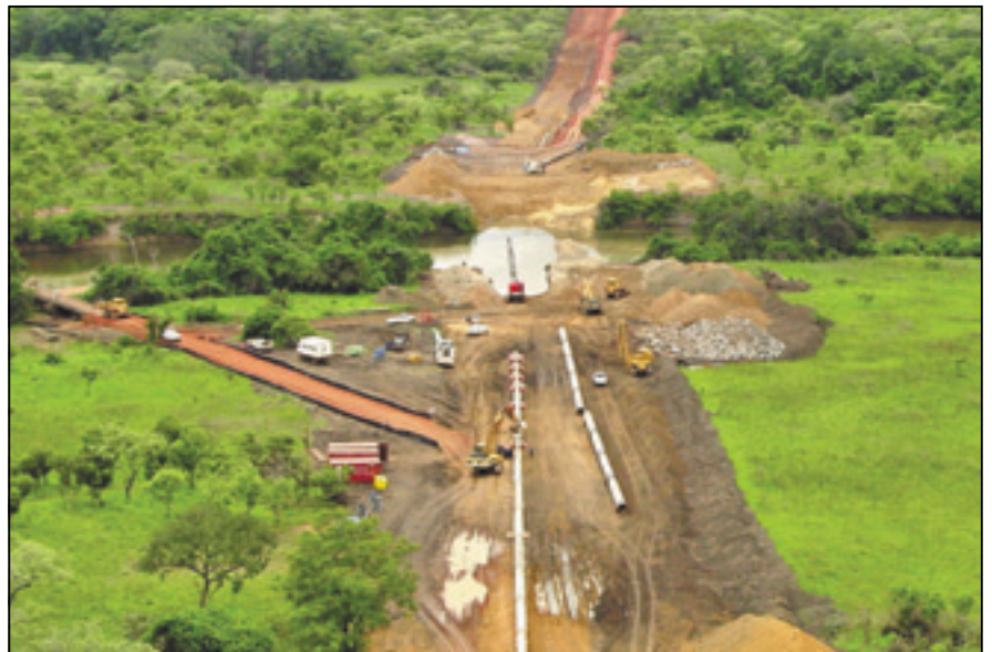
Plate 3.2 Example of a pipeline watercourse crossing with a shoo-fly road
