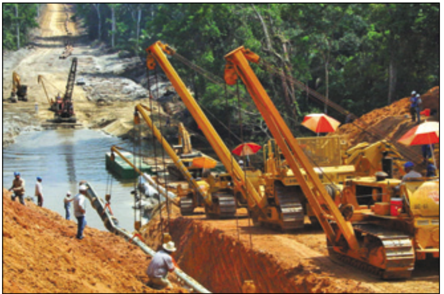
Plate 3.8 Example of a pipeline watercourse crossing
