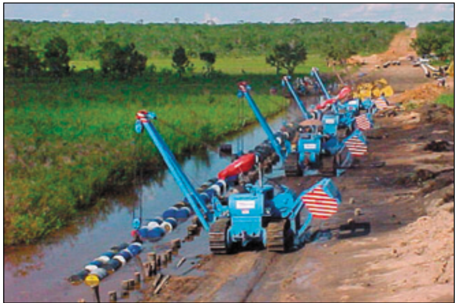
Plate 3.11 Example of a pipeline swamp crossing
