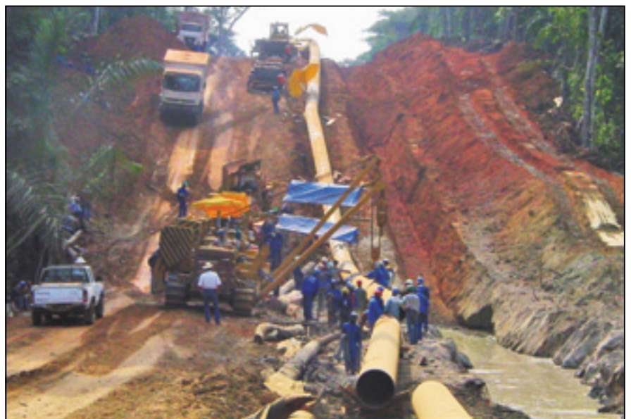
Plate 3.3 Example of a pipeline laying spread
