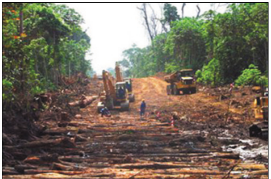
Plate 3.12 Example of timber riprap installation across a marsh area
