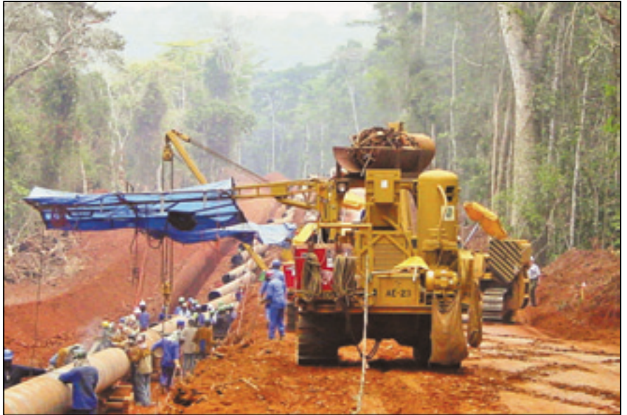
Plate 3.7 Example of pipeline spread stringing and welding pipe
