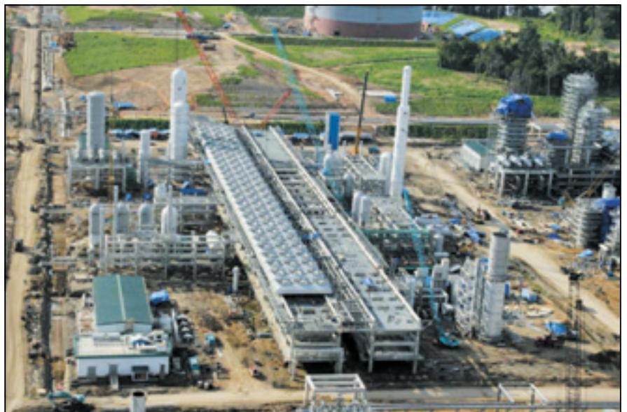
Plate 4.3 A process pipe rack 70% completed
