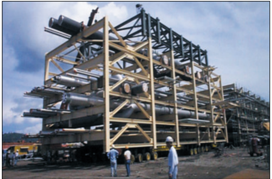
Plate 4.4 Typical pre-assembled pipe rack
