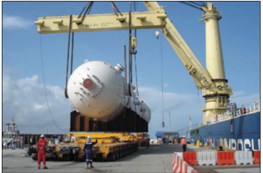
Plate 4.7 Amine absorber being unloaded
