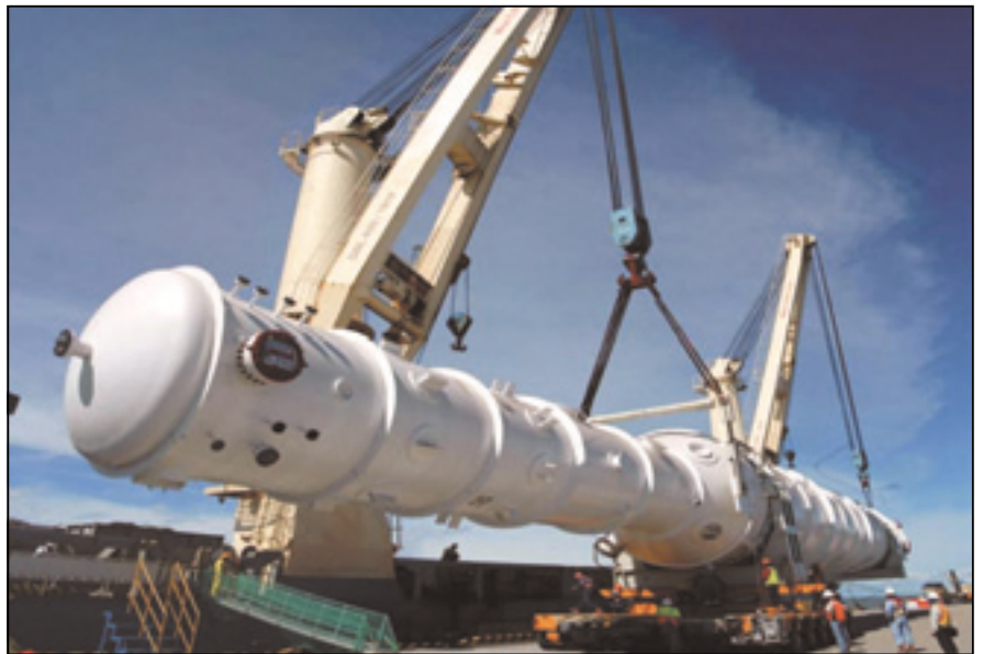
Plate 4.8 A cryogenic heat exchanger being unloaded
