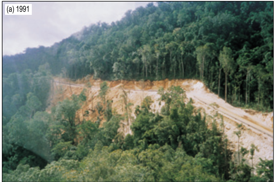
Plate 18.1 Regeneration of Kutubu to Kopi access way with cut and fill on ridge descending into Ai'io River
