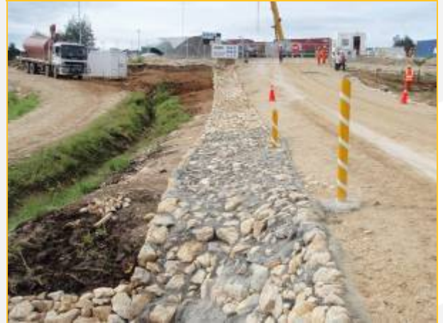
Plates 12.8 and 12.9: Silt catchment Oiyarip Camp construction
