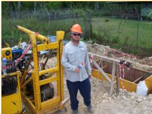
Plate 12.1: Preparation for drilling Moro Camp B water well
