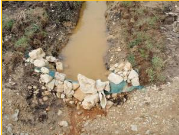
Plates 12.8 and 12.9: Silt catchment Oiyarip Camp construction
