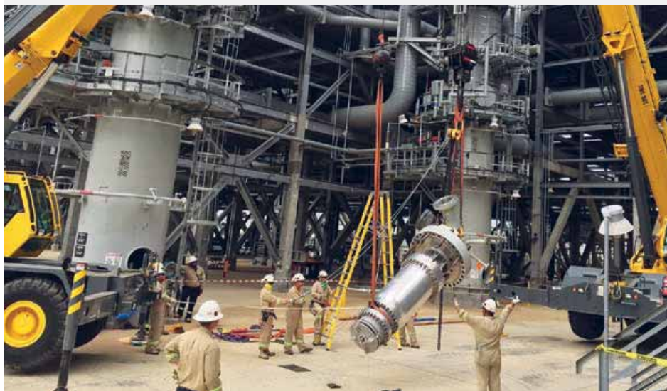
The turbine maintenance operation at the LNG Plant
