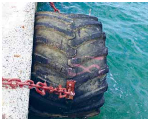
Plate 6.8 – Dump truck tyres donated to PNG Ports Corporation Limited being reused as wharf fenders
