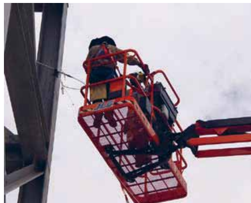
Third party specialists perform stack testing on the generator stack from a mechanical lift, to which they are harnessed
