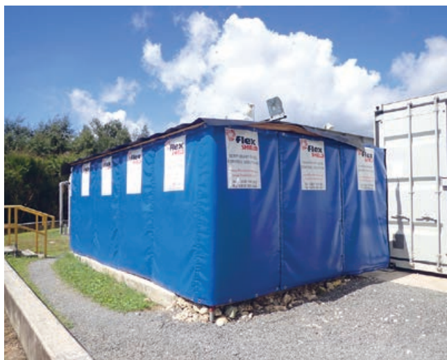
Noise barriers installed around the wastewater treatment plant at the HGCP
