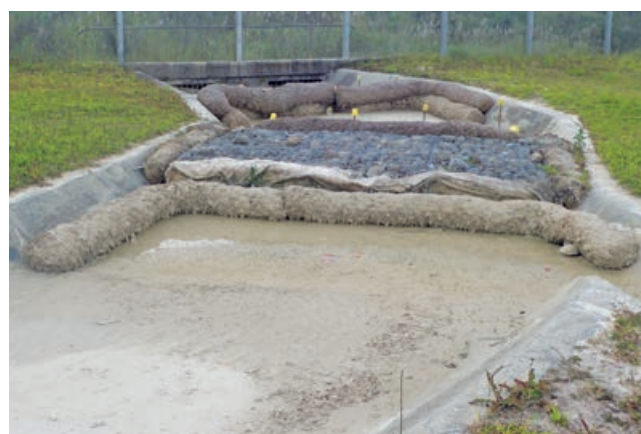
Sediment control devices installed in the stormwater drain at the HGCP
