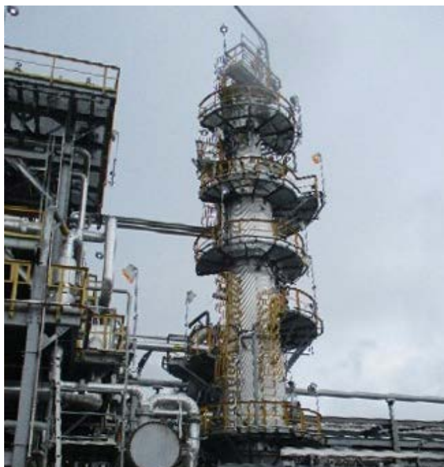
HGCP stabiliser column
