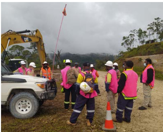
A toolbox talk prior to undertaking earthquake remediation works at KP 70
