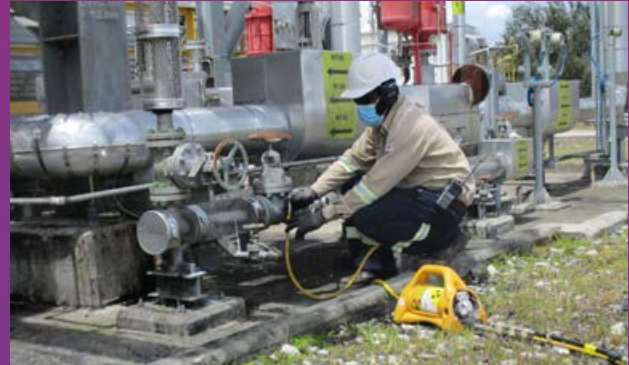
Nares Engineering Limited, Radiography Technician, Ken Wake, setting up digital radiography equipment for a pipeline inspection (above) and processing digital radiography images (below)
