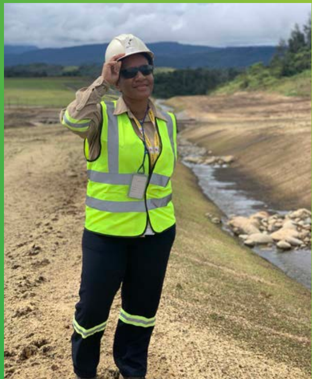
EMPNG Project Engineer, Denise Yakipu, at one of the recently constructed drains, which will help manage the impacts of rainfall in Komo
