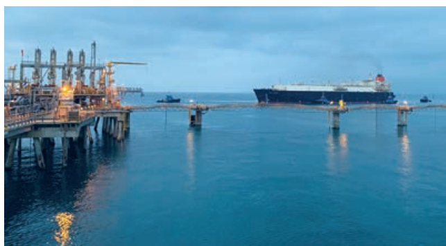
Long-term charter vessel Gigira Laitebo arrives at the LNG Plant Marine Terminal jetty to receive the 750 th LNG cargo
