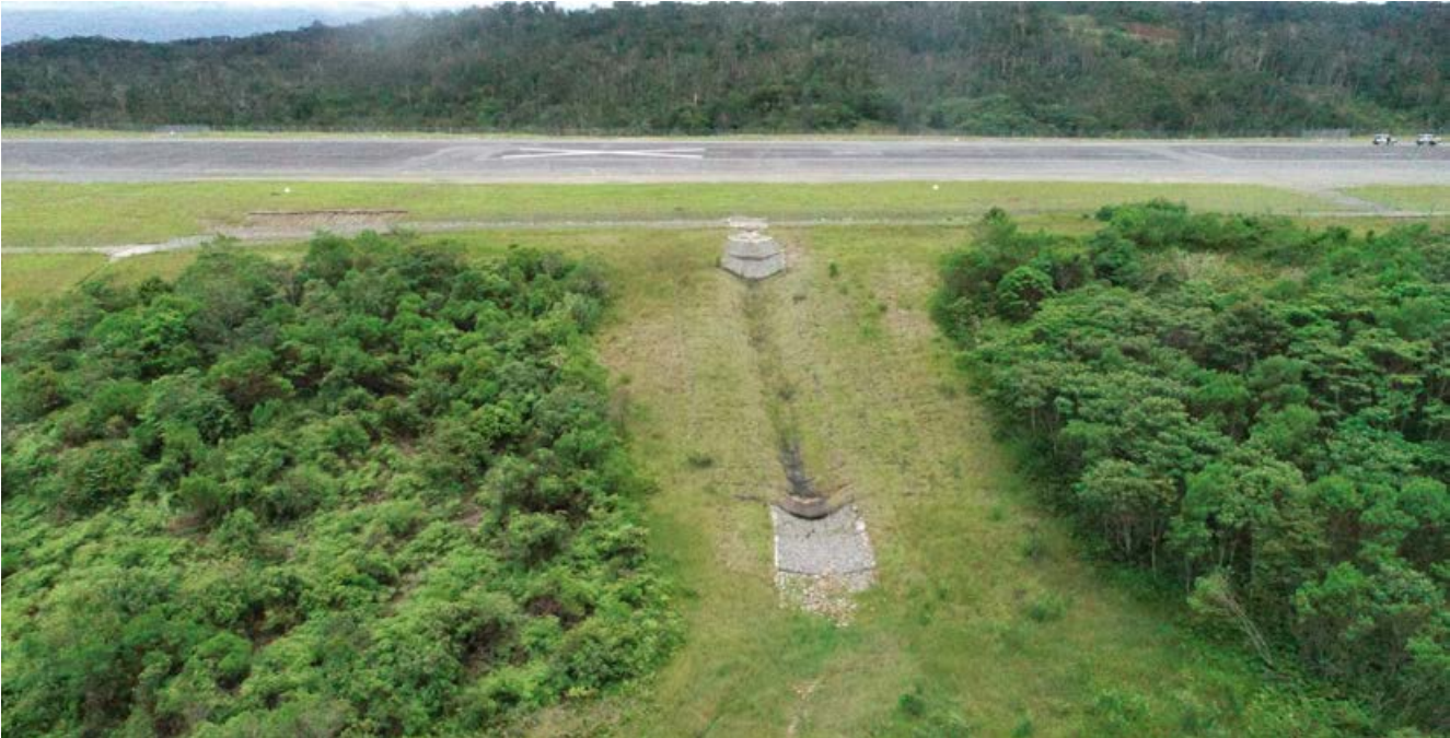
Revegetated stormwater drain at Komo Airfield
