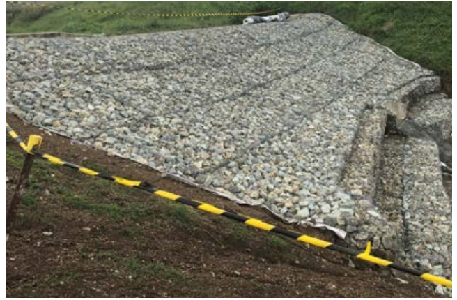
Completed embankment repair for the stormwater detention pond at ExxonMobil Haus
