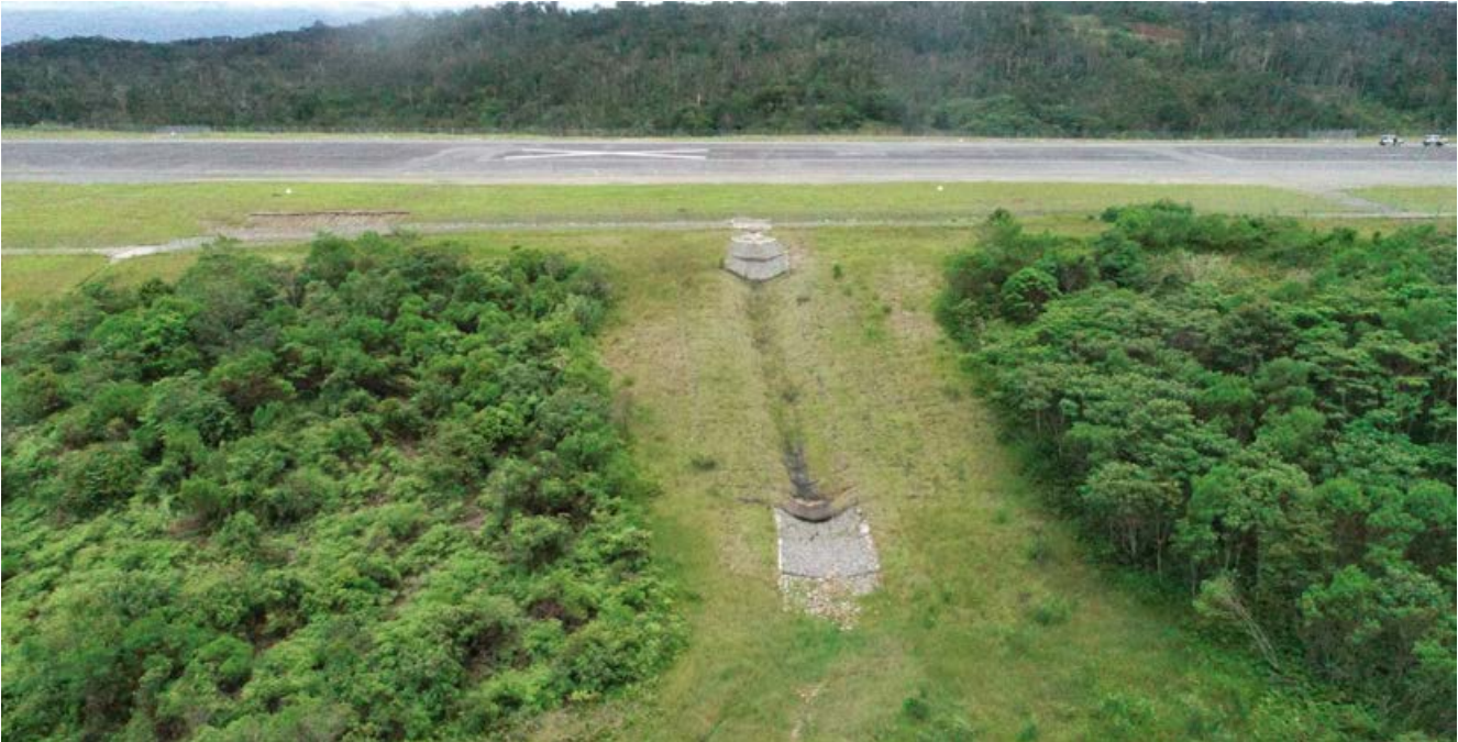
Revegetated stormwater drain at Komo Airfield
