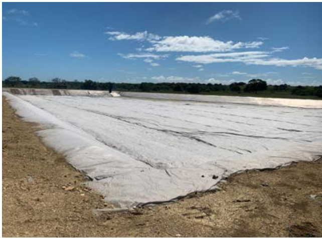
Landfill cell at the LNG Plant site being prepared for commissioning
