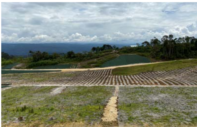
Native vegetation growing through jute matting at the Angore Wellpad C spoil fill area
