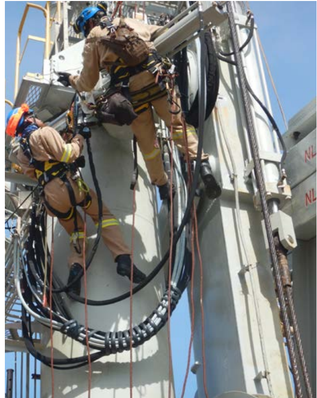
Hydraulic hose inspection and changeover is integral to the maintenance of the marine loading arm and requires rope access
