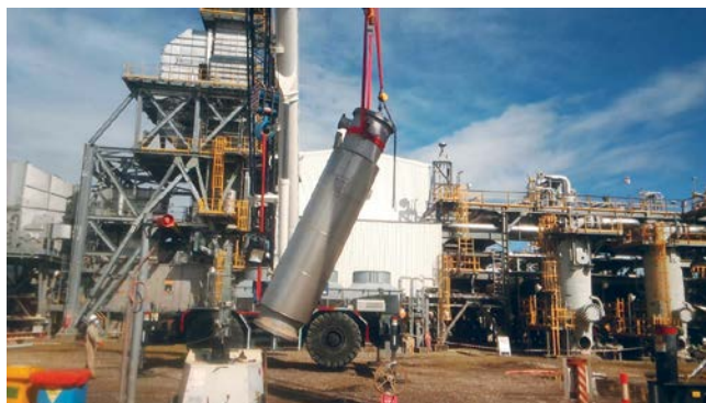
Removal of the HGCP monoethylene glycol regeneration package distillation column for cleaning
