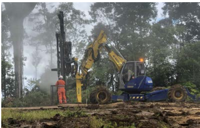
Installation of micropiles
