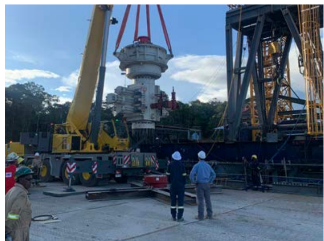
Blowout preventer installation at the Hides D1 well
