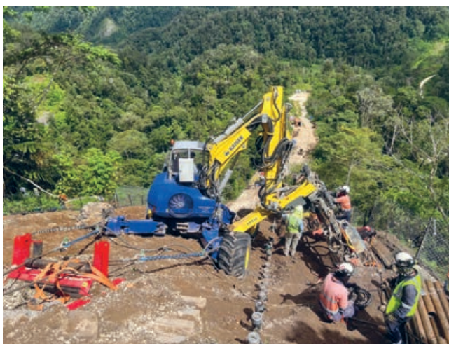
A 'spider' mobile walking excavator installing micropiles on a 37 degree incline
