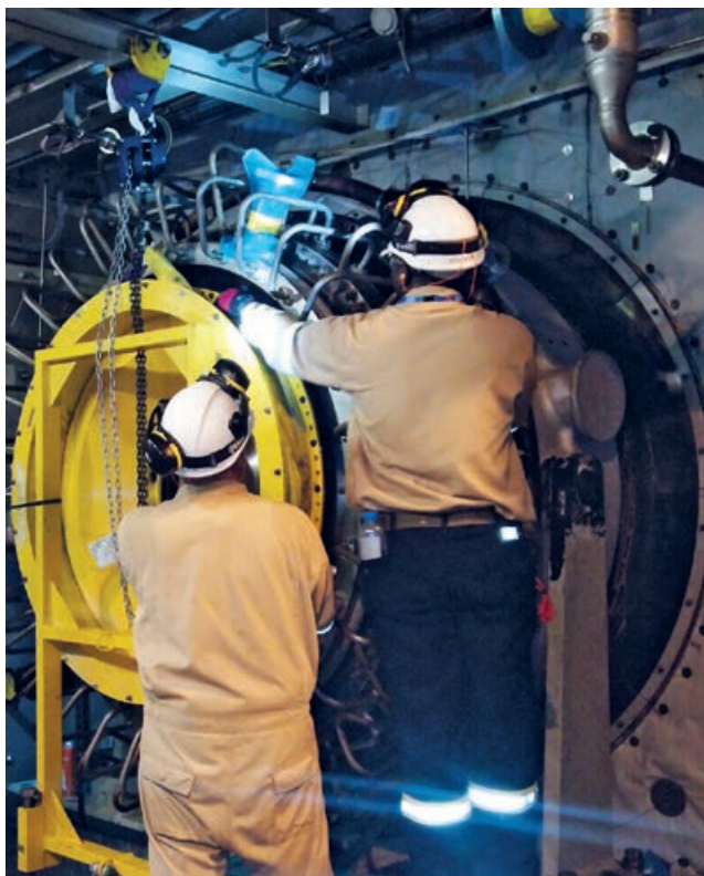
Workers undertaking maintenance on the LNG Plant Train 2 mixed refrigerant compressor turbine as part of the rate reduction scope
