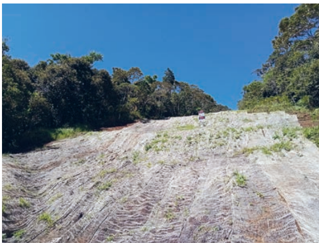
Geofabric installed along a steep section of the pipeline ROW to support native plant growth near the HGCP
