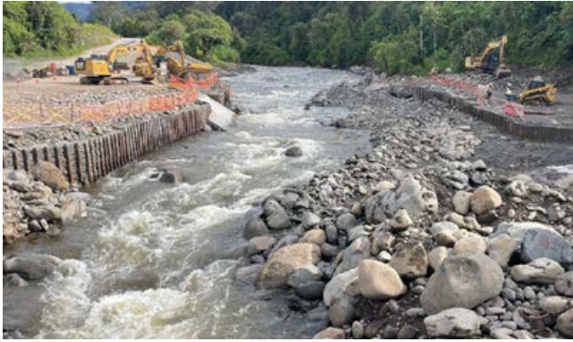
Progressive works on erosion, sediment control and reinstatement at the Mandali River crossing
