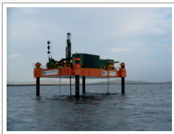
Plate 2.10 – Jack-up barge commencing soil boring at jetty head
