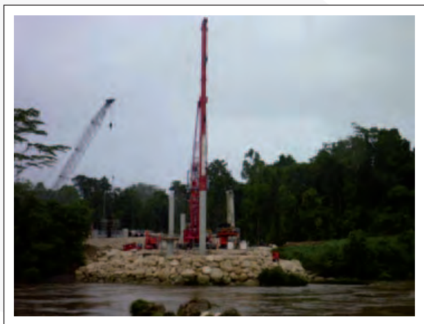
Plate 2.5 – Re-driving piles for the Kikori River Bridge
