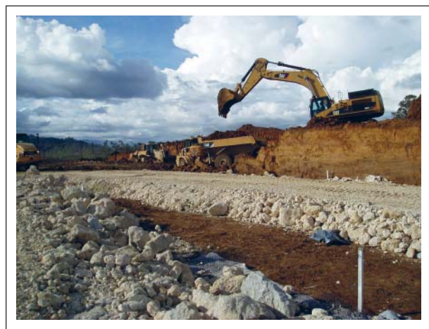
Plate 2.4 – Bulk earthworks for water bore pad at HGCP
