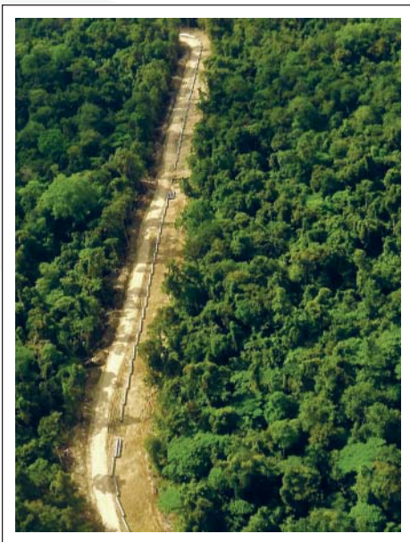
Plate 2.8 – Pipeline stringing at Kilometer Point 268
