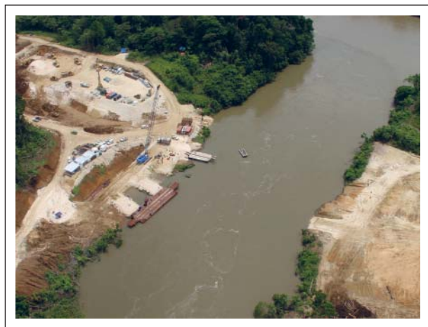
Plate 2.4 – Bulk earthworks for water bore pad at HGCP
