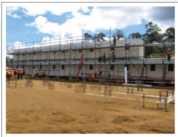
Plate 2.5 – Main camp accommodation unit assembly
