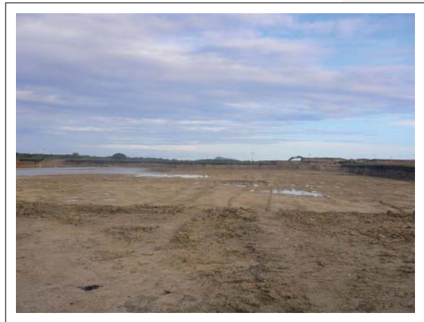
Plate 11.4 – Example of a sediment basin used for erosion control
