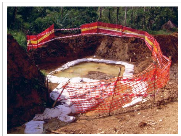
Plate 11.4 – Example of a sediment basin used for erosion control
