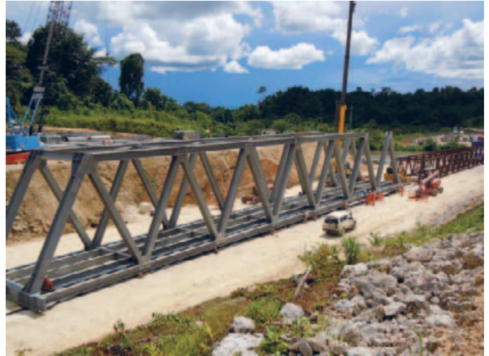
Plate 2.2 – Mubi River Bridge truss assembly
