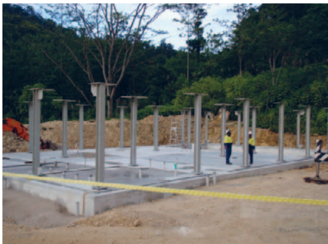
Plate 2.9 – New Central Control Room foundations at the Kutubu Central Processing Facility
