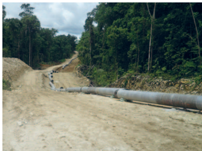
Plate 2.5 – Pipeline stringing
