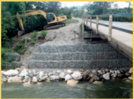
Bridge abutment reinforcement at Darmena Creek Bridge
