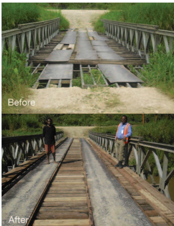
Plate 5.11 – Det Bridge before and after resurfacing
