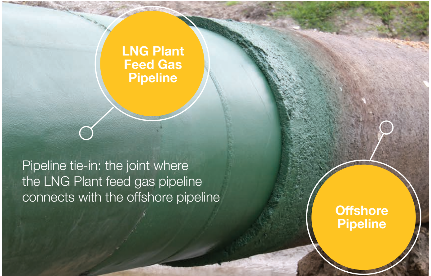
Tie-in between the LNG Plant feed gas pipeline and the offshore pipeline prior to backfilling
