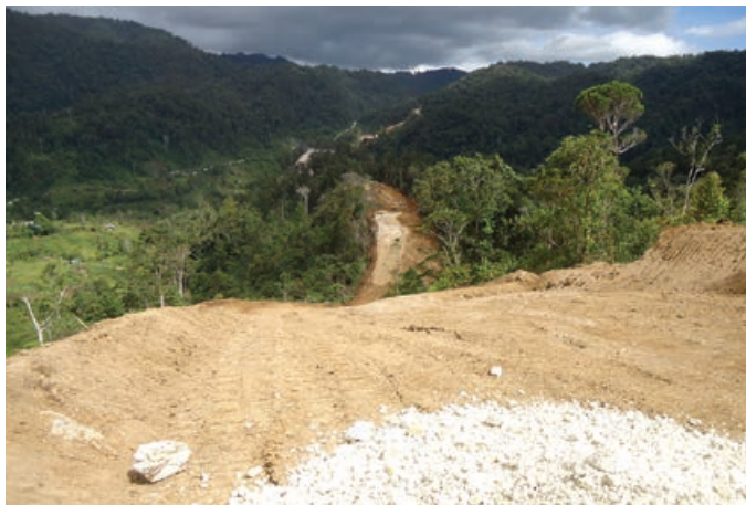
Clearing and grading activities along the reduced ROW width between Kilometre Points 64 and 65
