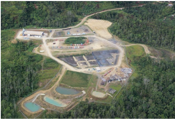
Hides Waste Management Facility showing completed landfill cells
