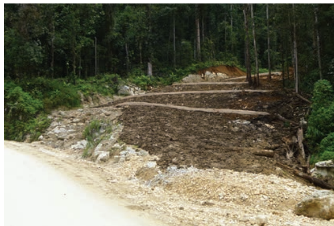
Reinstatement and installation of erosion control berms on the Kutubu Spurline from the Kutubu Central Processing Facility bypass road
