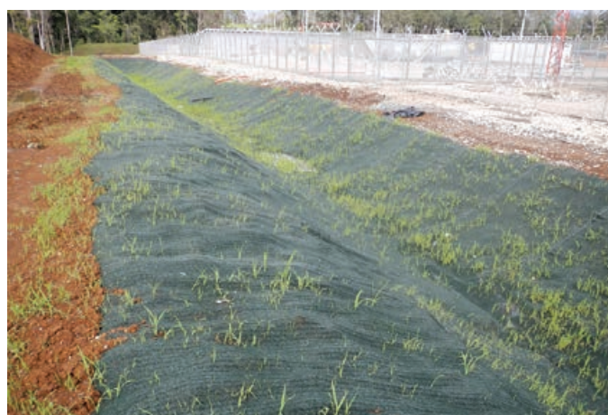
A reinstated area following topsoil spreading, seeding and application of turf reinforcement mat
