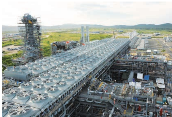
Completed painting on Train 2 and insulation on Main Cryogenic Heat Exchanger prior to handover
