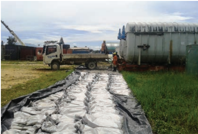
Preparing the wastewater treatment plant at Moro Camp 5 for demobilization by removing, bagging and drying sludge for incineration
