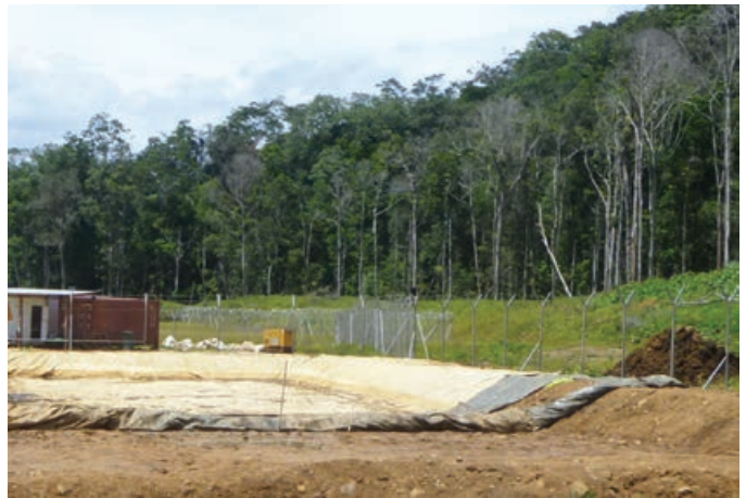
Rolling of liner for reuse during decommissioning of the fuel storage bund at Awatangi Quarry Camp 7
