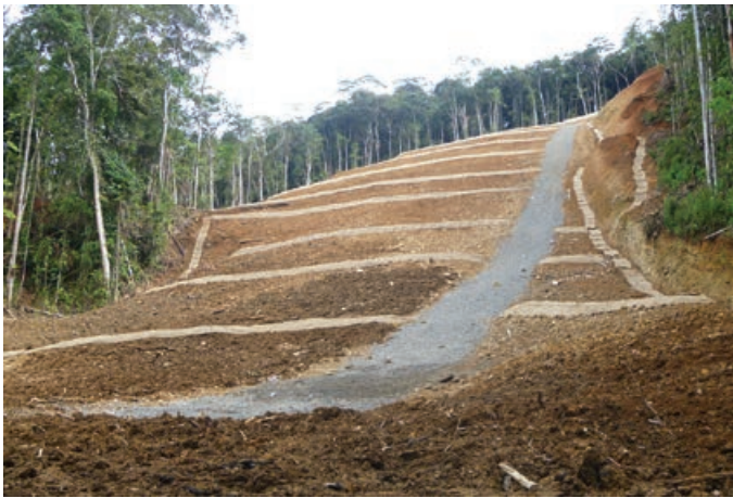
Reinstatement of the Tagari Fault Crossing at Kilometre Point 6.3 of the onshore pipeline
