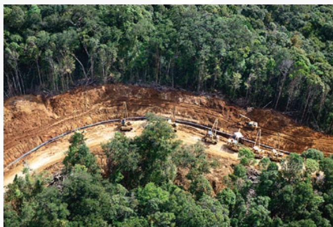
Lowering-in of the onshore pipeline
