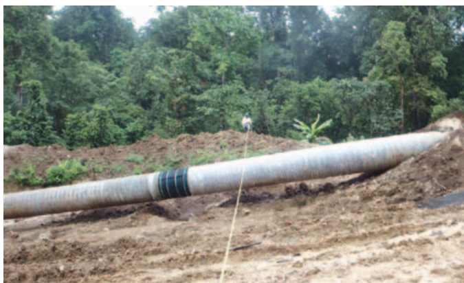
Plate 10.1 – Verifying the ROW width after cutting and grading activities
