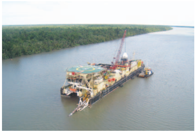
Plate 2.2 – Pipelay barge laying the shallow water section of the offshore pipeline
