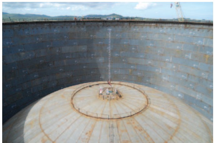
Plate 2.3 – Roof of the north LNG tank being air raised
