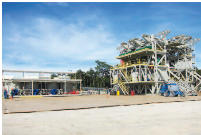
Plate 9.1 – Portable interlocking matting at drilling site minimizes dust
