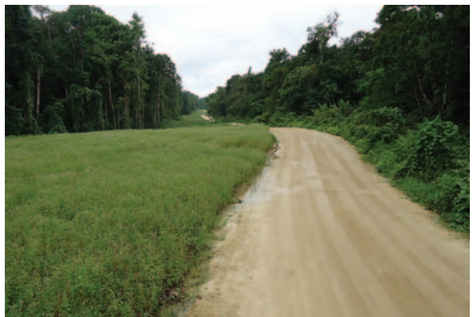
Plate 10.7 – Onshore pipeline ROW eight weeks after final reinstatement between Kilometre Point 193 and 226
