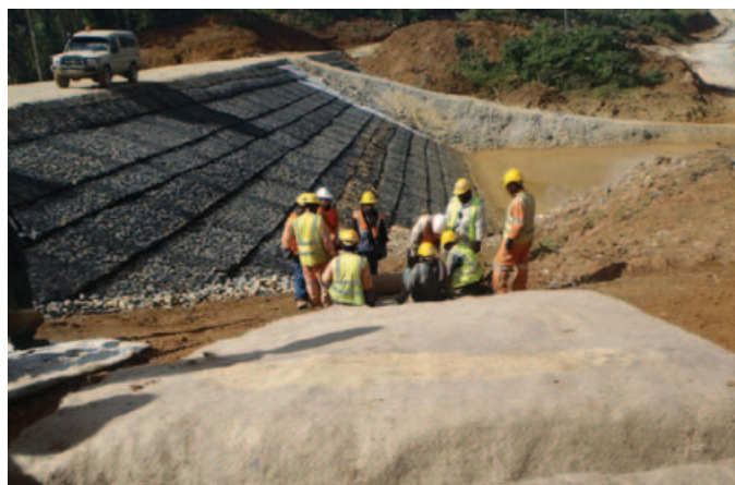
Plate 11.4 – Erosion control measures showing rock check, jute matting and sediment retention dam
