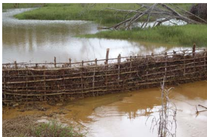
Plate 11.5 – Silt fence made from site-sourced vegetation at the Komo Airfield
