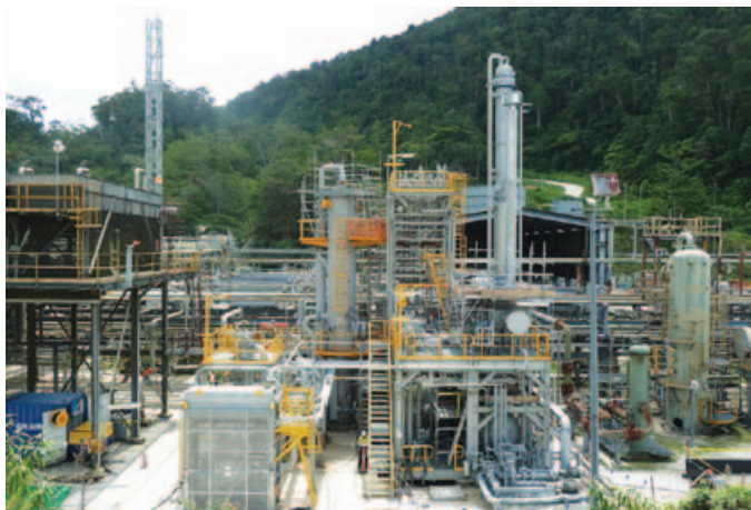
Plate 2.5 – Commissioned triethylene glycol unit at the Kutubu Central Processing Facility
