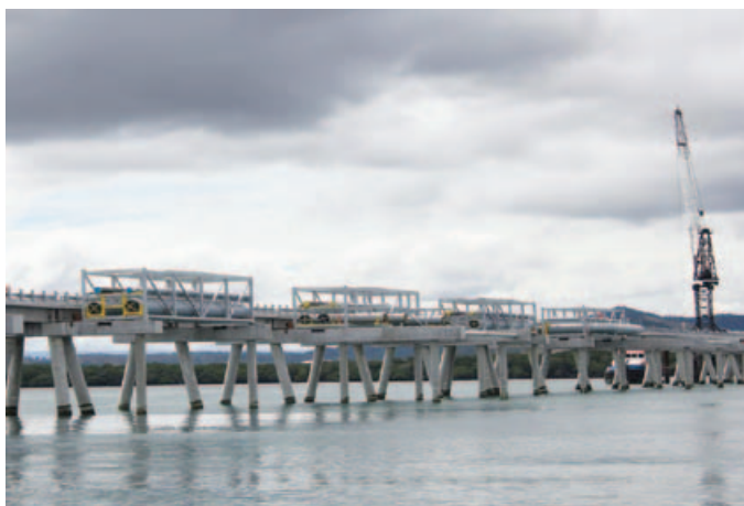
Plate 2.4 – Piperack modules in place on the jetty trestle
