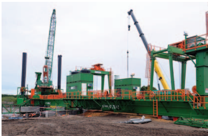
Plate 2.6 – Marine jetty piling
