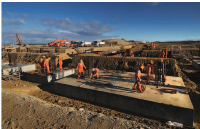
Plate 2.7 – Construction of LNG Plant process pipe rack
