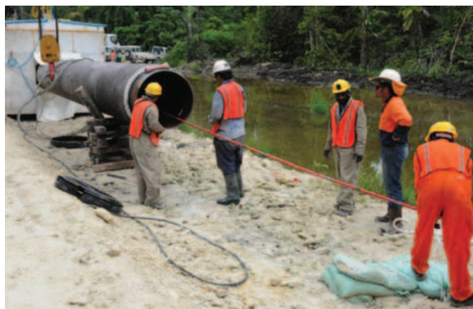
Plate 2.4 – Pipe welding
