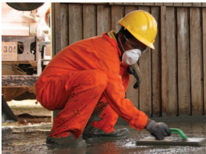
Plate 5.10 – Trainee laying a new concrete floor at the Boera Elementary School
