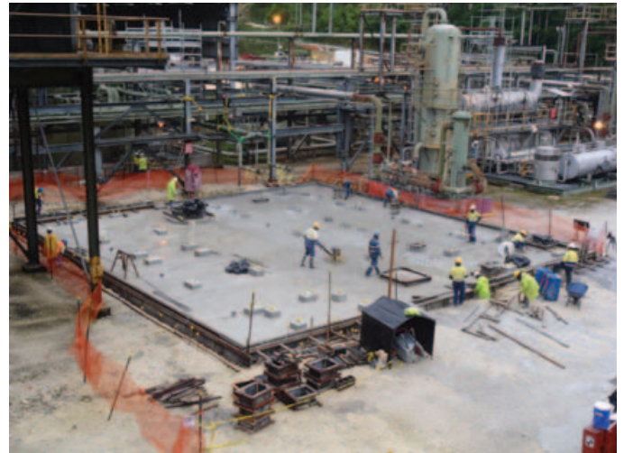
Plate 2.8 – Footings for the Kutubu Central Processing Facility dehydration unit
