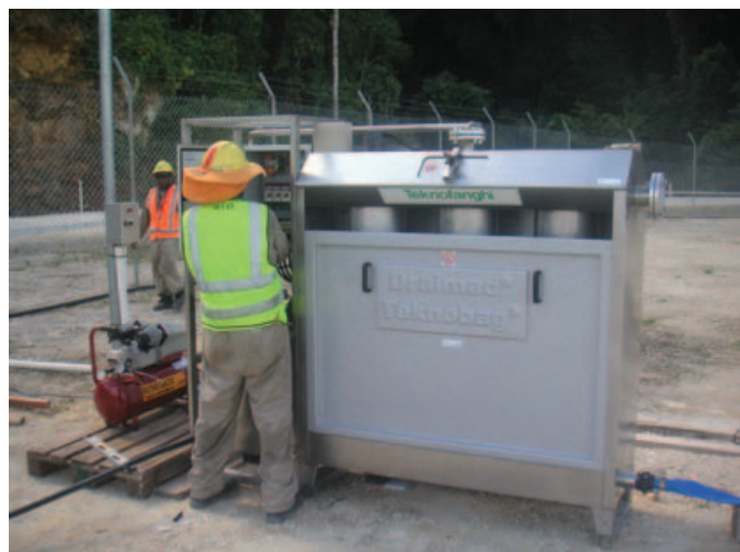
Plate 9.4 – Preparation of sludge drying machine to treat sludge from demolished Kopi Scraper Station Bush Camp wastewater treatment plant
