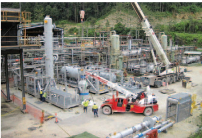
Plate 2.4 a-b – Triethylene glycol package installation at the Kutubu Central Processing Facility
