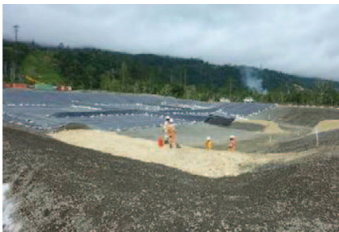
Plate 9.2 – Hides Waste Management Facility under construction showing grey lined landfill cell
