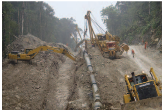
Plate 2.3 – Pipe lowering-in activities at Kilometre Point 253
