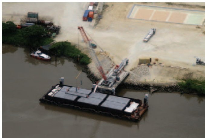
Plate 2.1 – Final line pipe delivery being offloaded from the pipe barge at Kopi Shore Base
