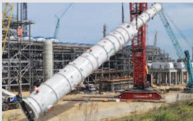
The MCHE being lifted into place on Train 2
