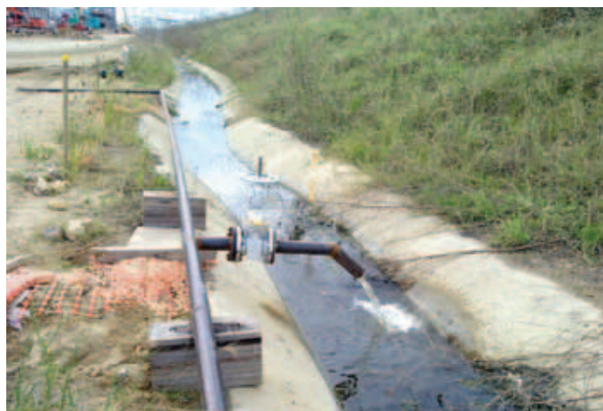
Plate 11.1 – Hydrotest water at the LNG plant site being discharged into a concrete drain and finally into the main LNG plant site sedimentation pond
