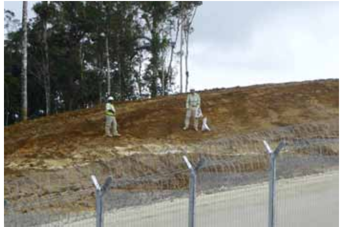
Plate 10.6 – Casting seeds on the HGCP perimeter road batter
