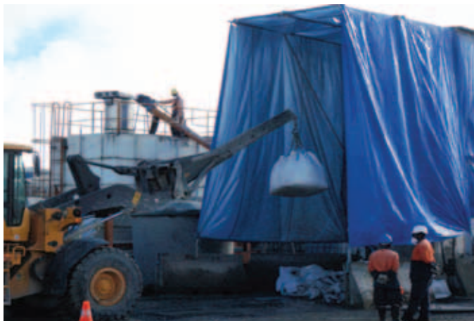
Plate 9.1 – Minimizing dust by delivering cement bags directly into the shrouded area
