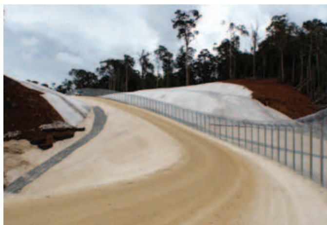
Plate 11.3 – North-eastern boundary of the HGCP site showing erosion control matting, green seeding, silt fencing and a rock lined drain to a culvert
