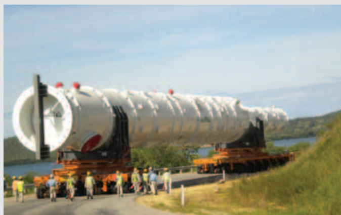
The MCHE on self-propelled modular transports enroute to the LNG plant site
