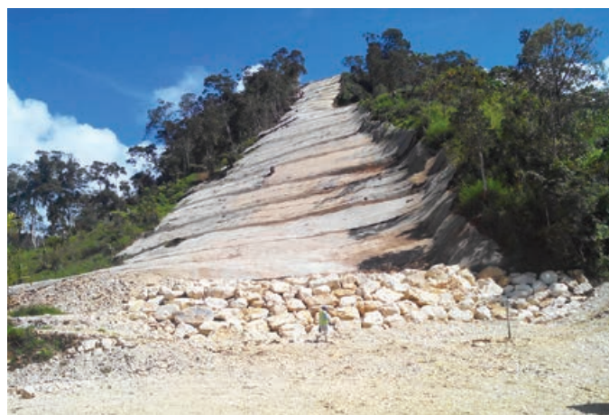
Extensive erosion control measures applied to steep slopes
