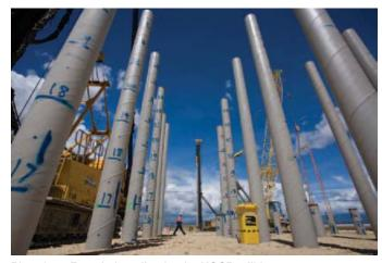
Plate 2.1 – Foundation piles for the HGCP utilities area
