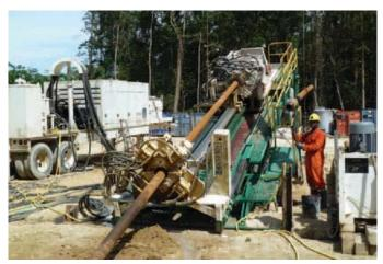
Plate 2.3 - Horizontal directional drilling rig in operation
