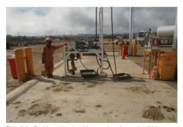
Plate 9.8 - Fuel farm showing drip trays, bunding and spill kits
