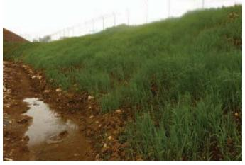
Plate 11.2 – Stabilization of batter slope using Japanese Millet *Echinochloa* spp. at Komo Main Camp
