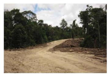
Plate 10.4 – A ROW section spread with topsoil as part of reinstatement
