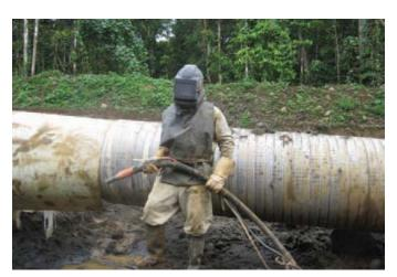
Plate 7.5 - Worker conducting abrasive blasting
