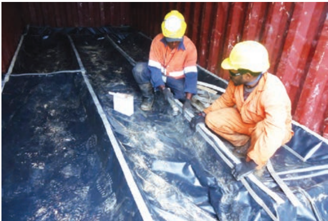
A segmented bund used to store waste before transfer to off-site disposal facilities
