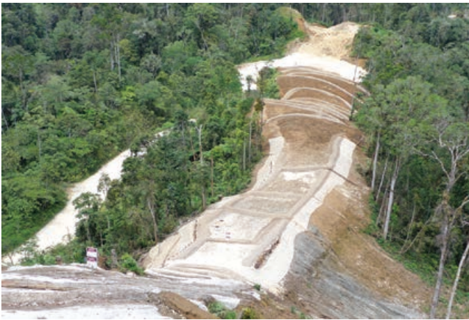
Erosion control and slope stabilization along the pipeline
