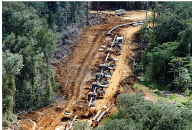
Automatic welding on the final sections of the main onshore pipeline
