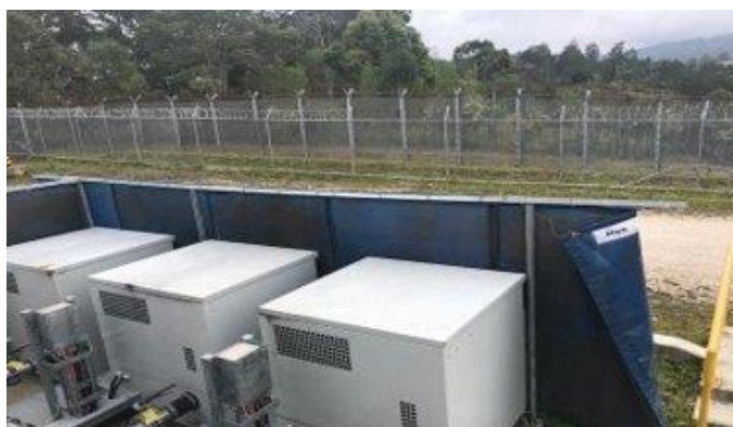
Figure 4.4: Noise Barriers being Replaced at HGCP
