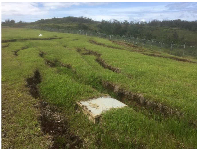
Figure 4.6: Komo Airfield Apron in Area Constructed over Fill
