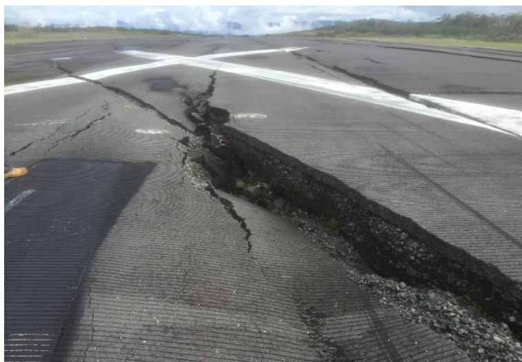
Figure 1.2: Example of Earthquake Damage to fill Portion of Komo Airfield
