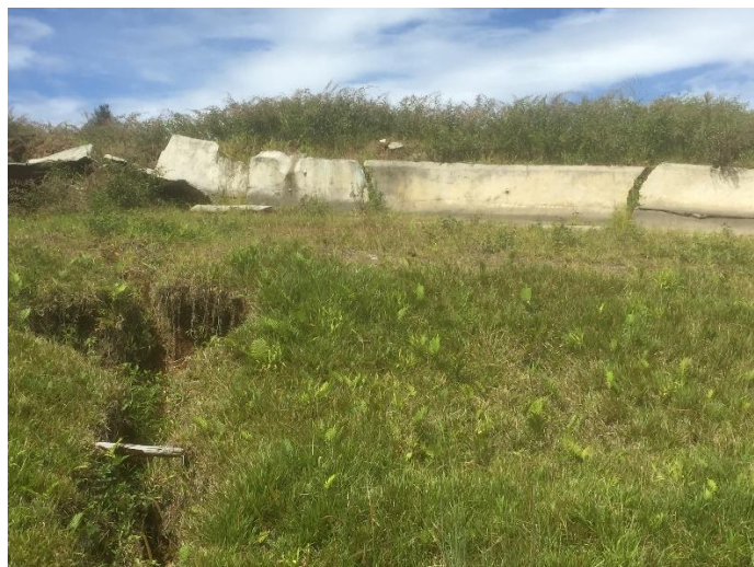
Figure 4.5: Drainage Infrastructure at Komo Airfield Destroyed by the Earthquake
