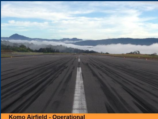
Komo Airfield - Operational
