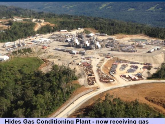
Hides Gas Conditioning Plant - now receiving gas
