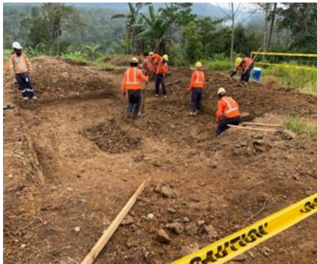
Figure 4.4: Installing Drainage at KP6
