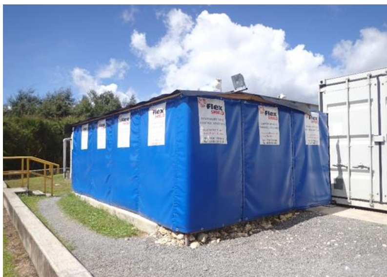
Figure 4.3: Final Noise Barriers at HGCP WWTP Blower Enclosure
