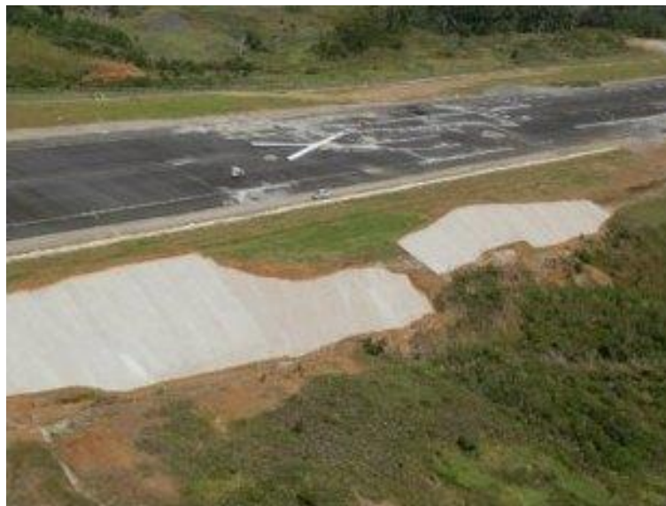
Figure 1.1: Repairs to Earthquake Damage at Komo Airfield
