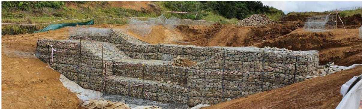
Figure 4.10: Zone 1 - Sediment Retention Structure
