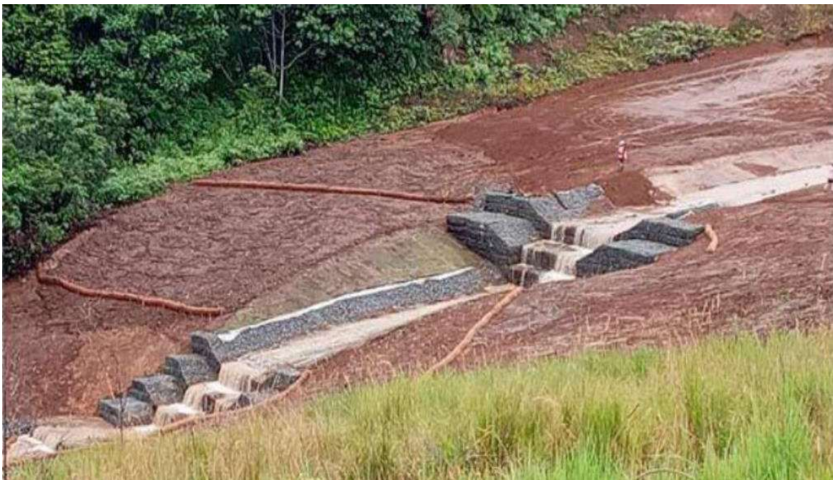
Figure 4.11: Zone 1 Drain 5 Completed
