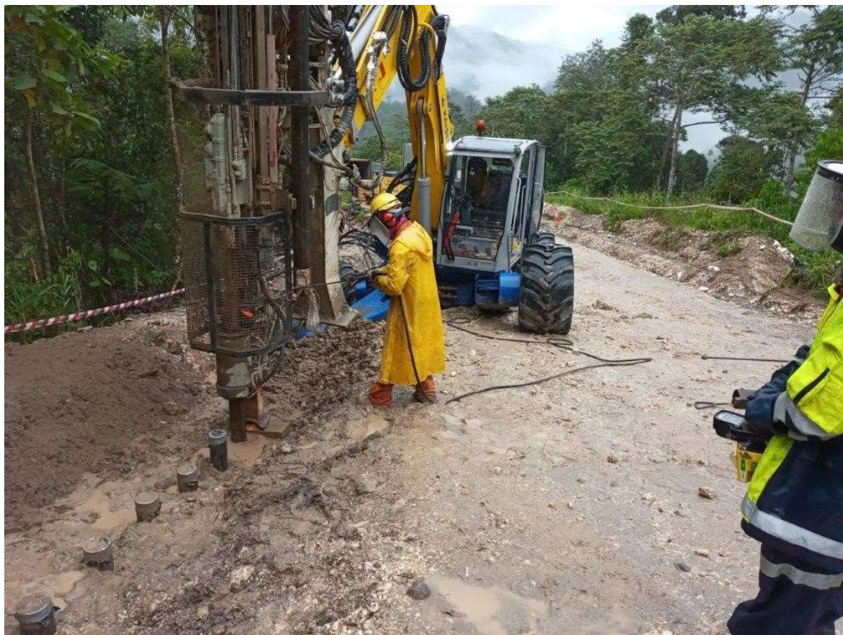
Figure 1.3: ROW Stabilization – Installing Micropiles at KP 64.5
