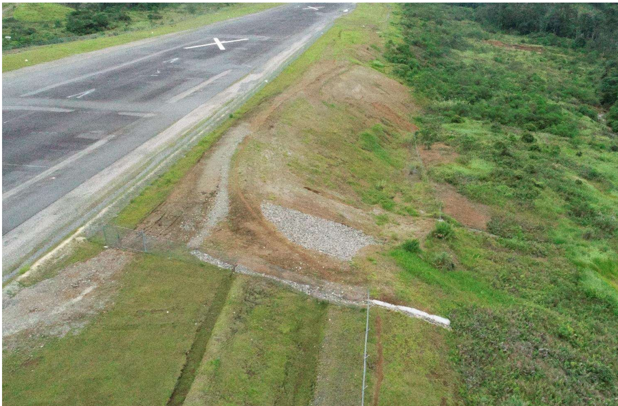
Figure 4.12: Zone 2 Landslip Stabilization
