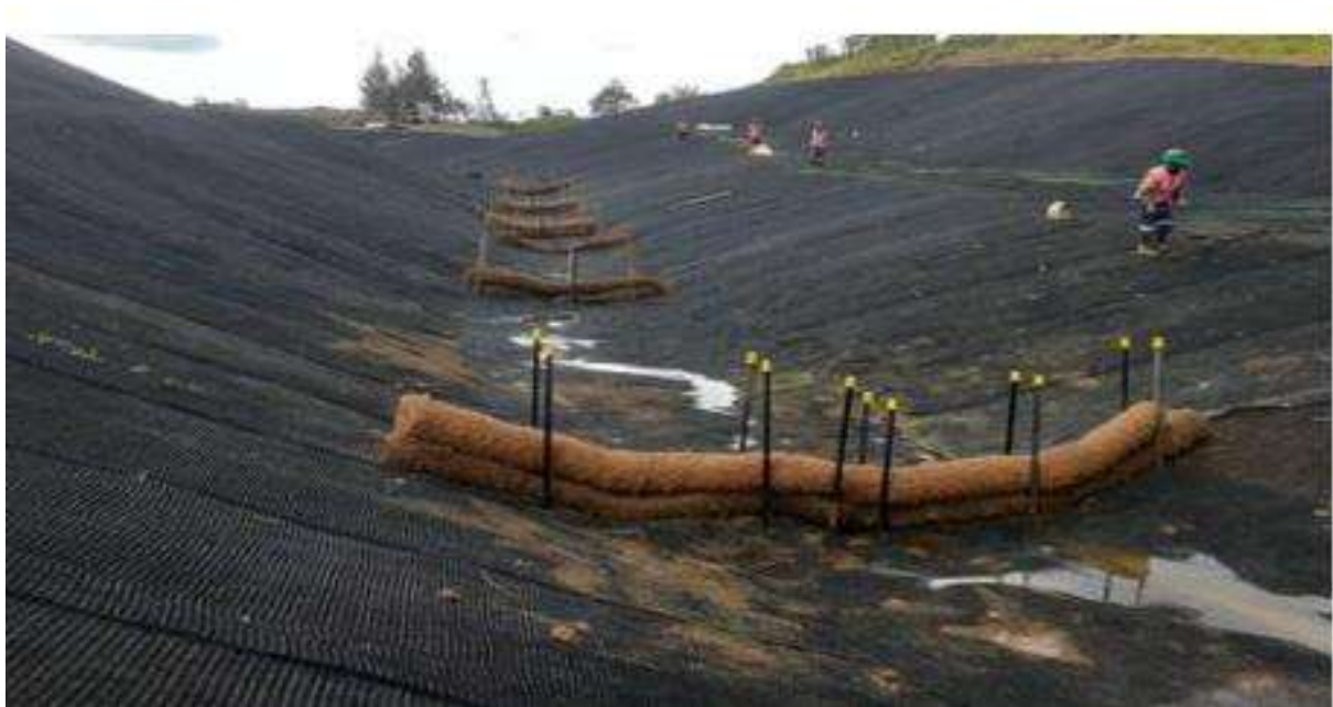
Figure 4.14: Zone 3 Drain 18 under Construction
