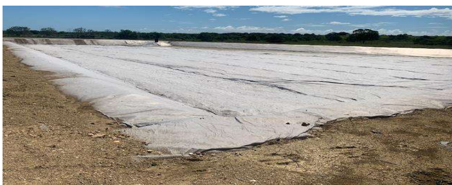
Figure 4.3: New Liner at Construction Landfill Cell C
