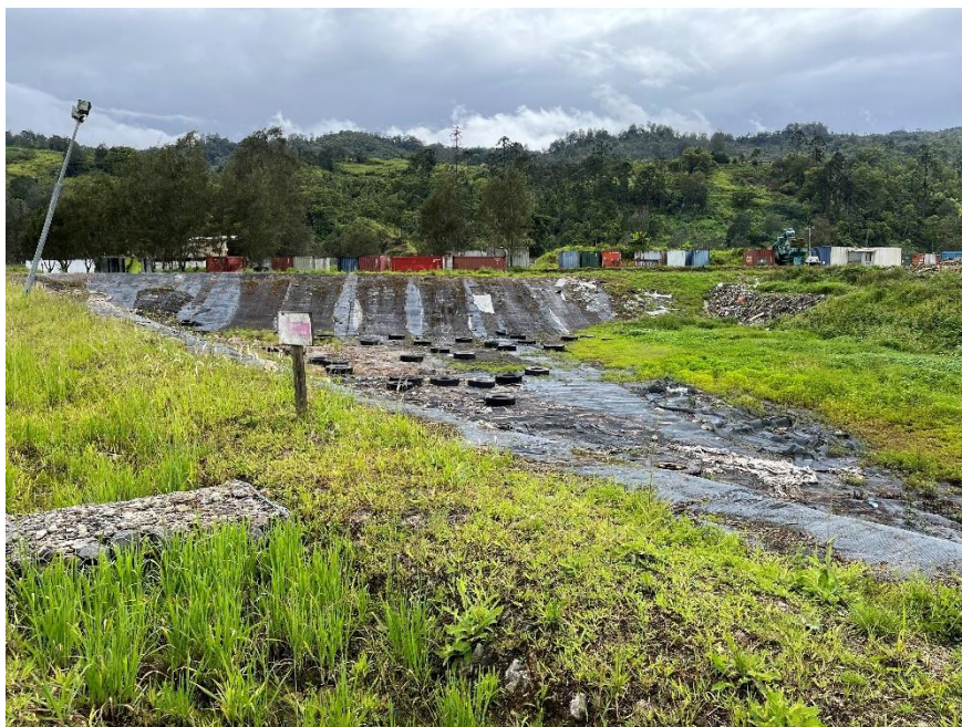
Figure 4.2: Exposed Landfill Liner at HWMF
