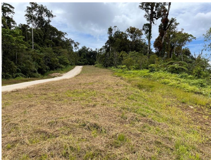
Figure 4.13: ROW Stabilization at KP 82 after Reinstatement
