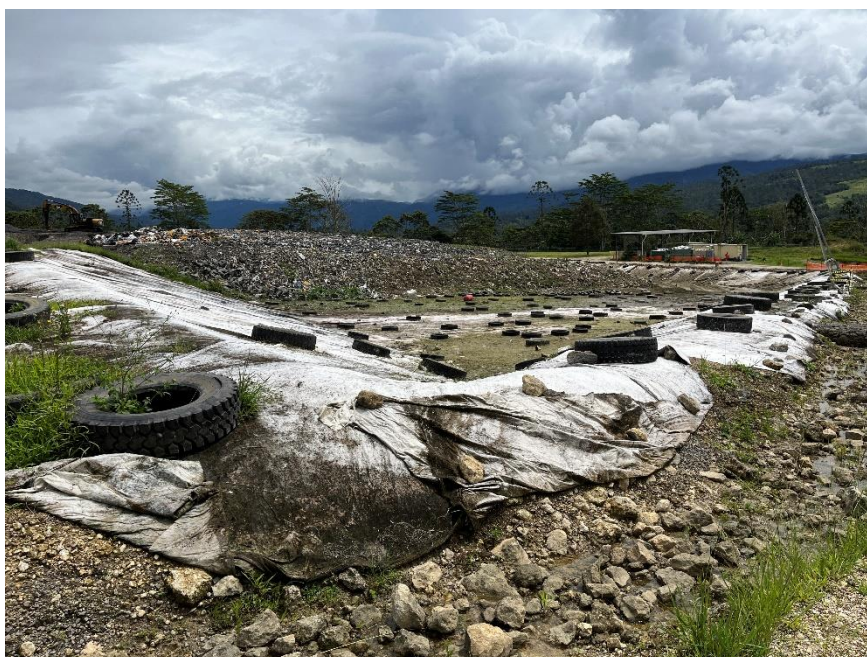
Figure 4.2: Geosynthetic Cover over Landfill Liner at HWMF
