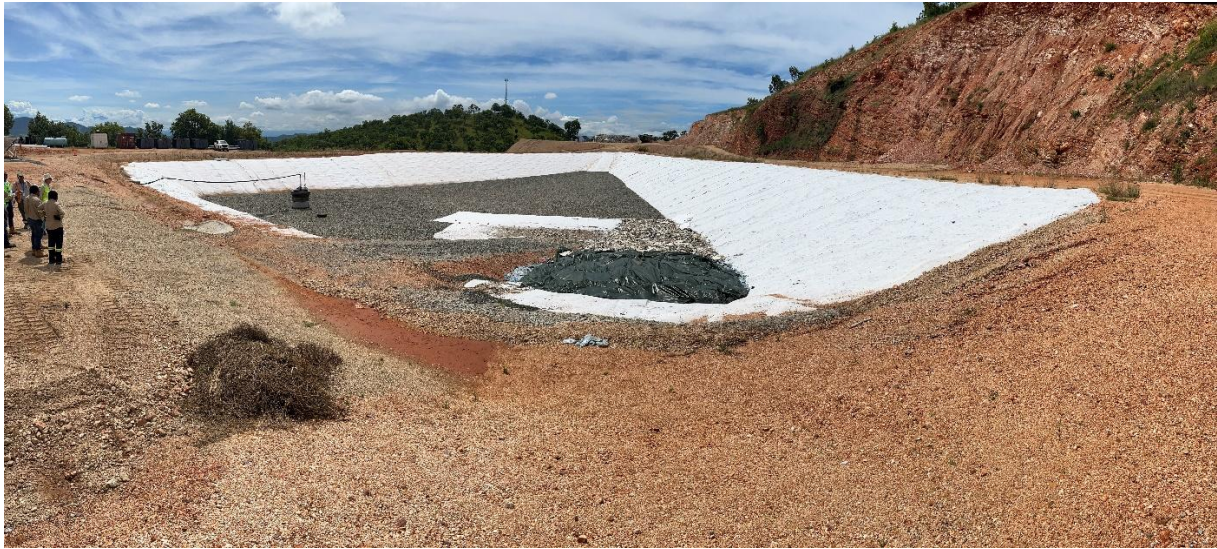
Figure 4.3: TWM Engineered Landfill Starting to Accept Waste
