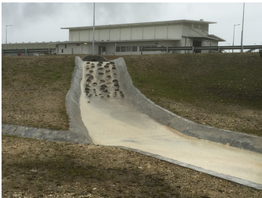
Figure 4.3: New E&S controls at the HGCP
