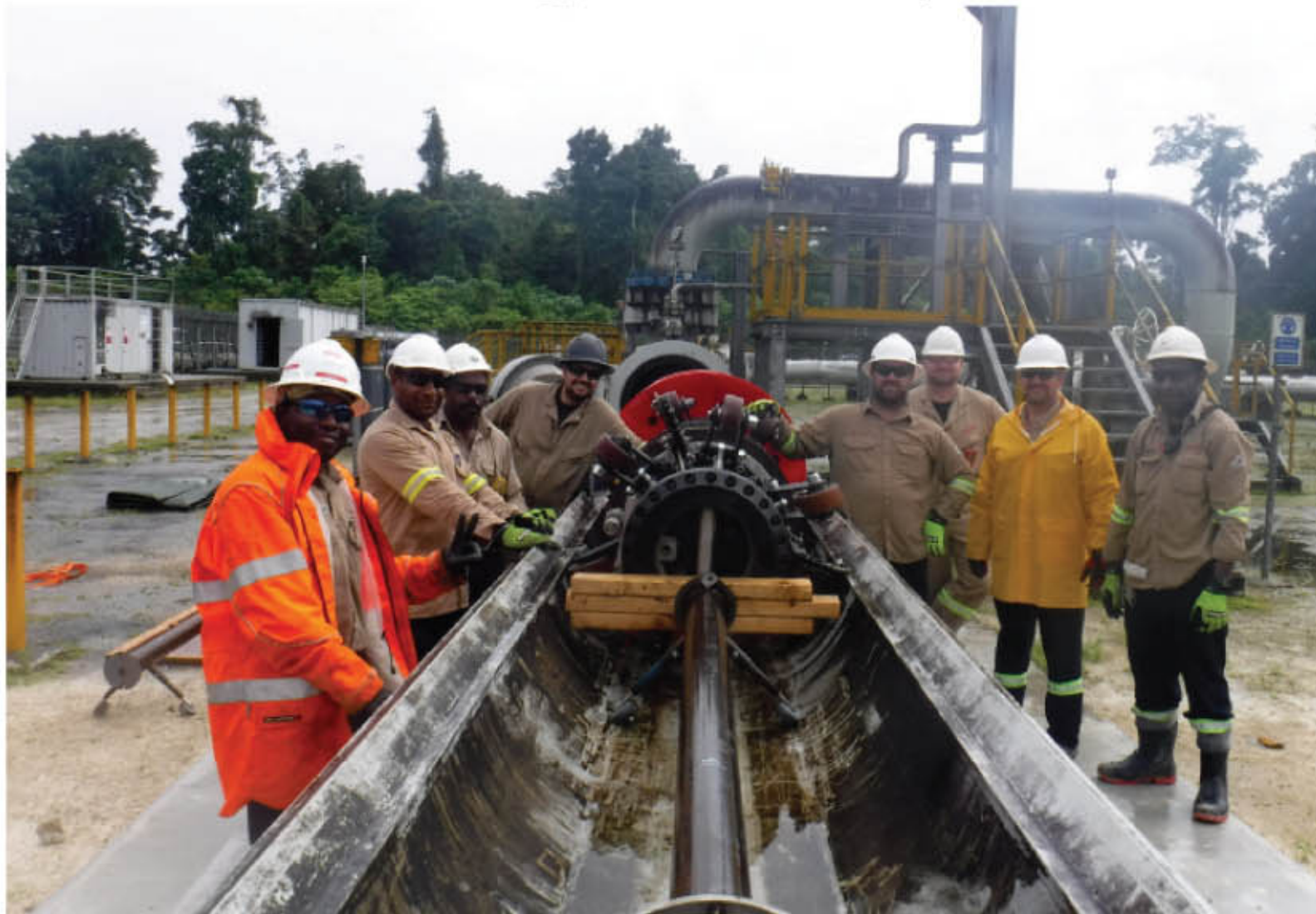
Maintenance crew launching the PIG at the Kopi Scraper Station in Hela Province.
