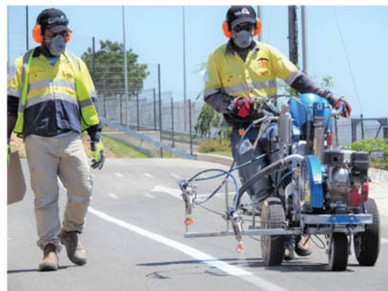
Justin Simon working the line marking machine with Alus Timbiyu assisting him as they repainted the markings on the internal roads and carpark within the ExxonMobil PNG Head Office compound.
